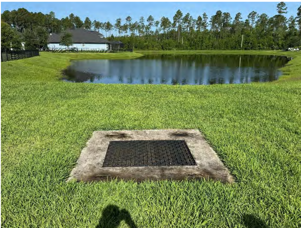
Beacon Lake Phase 2A – SMF 17 Control Structure (05-29-2026)
