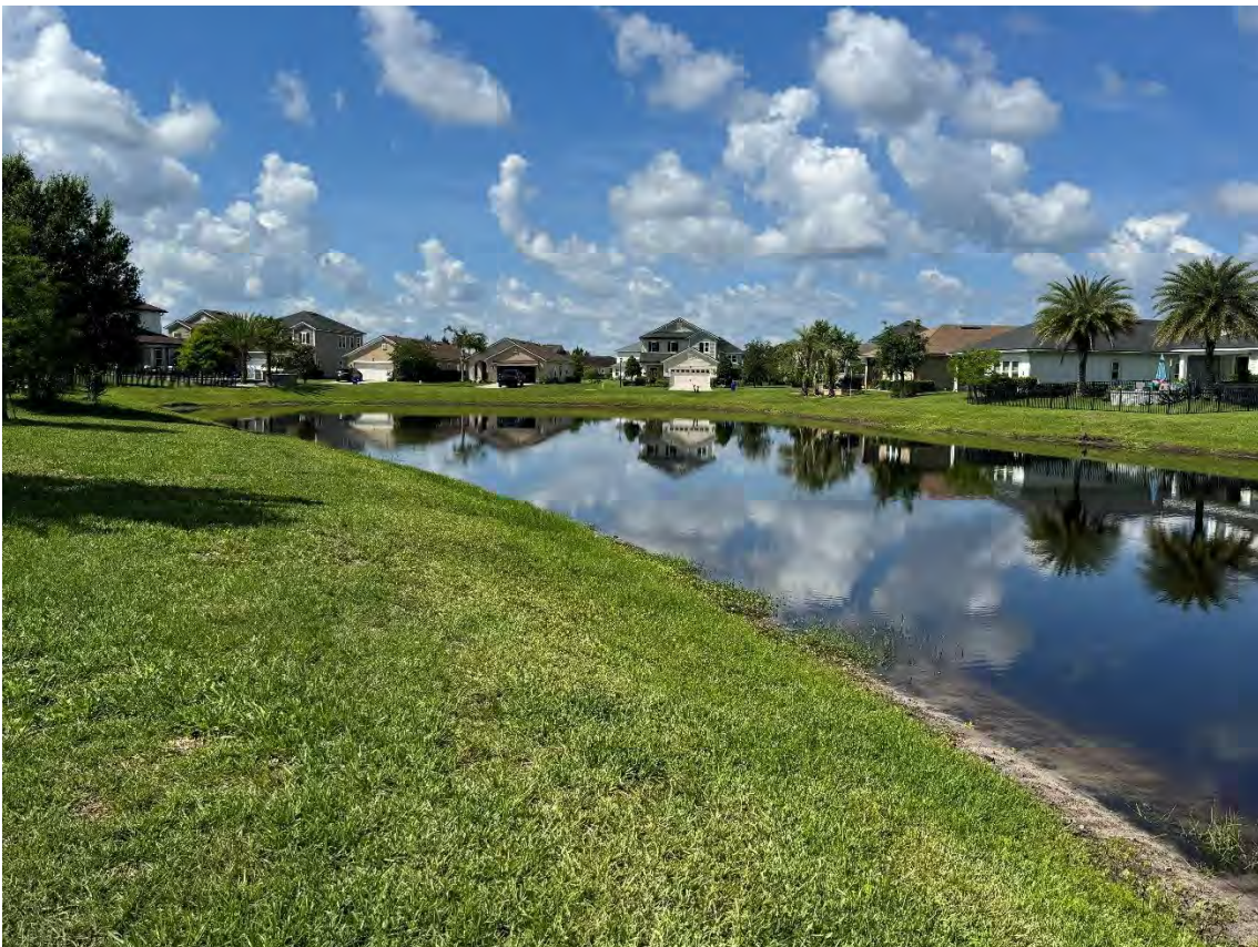
Beacon Lake Phase 1 – Storm Water Management Facility 15 (05-21-2026)
