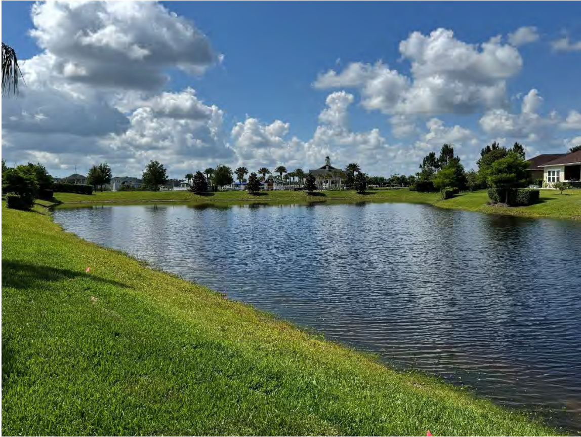
Beacon Lake Phase 1 – Storm Water Management Facility 16 (05-21-2026)
