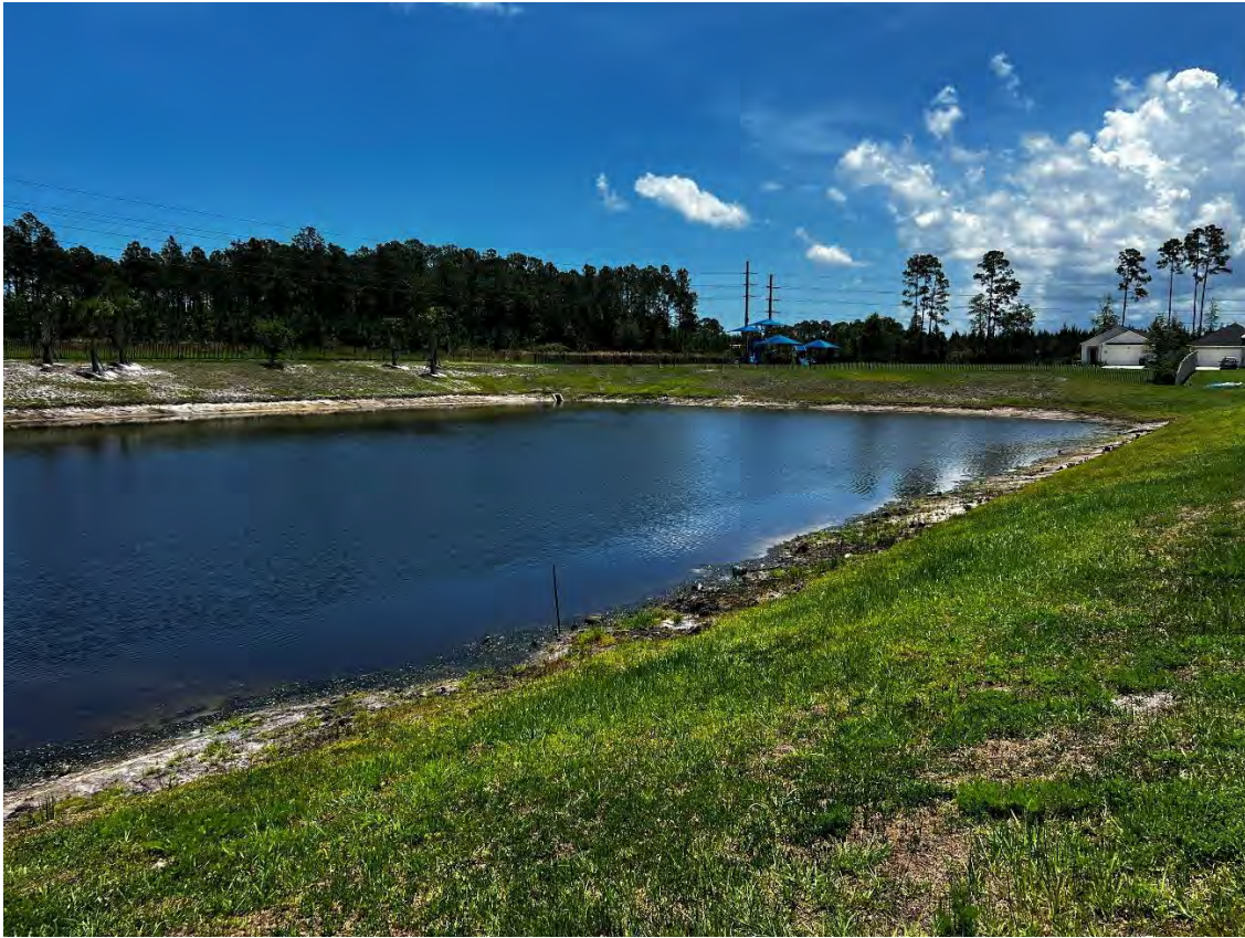
Beacon Lake Phase 4 – Storm Water Management Facility 25 (05-21-2026)
