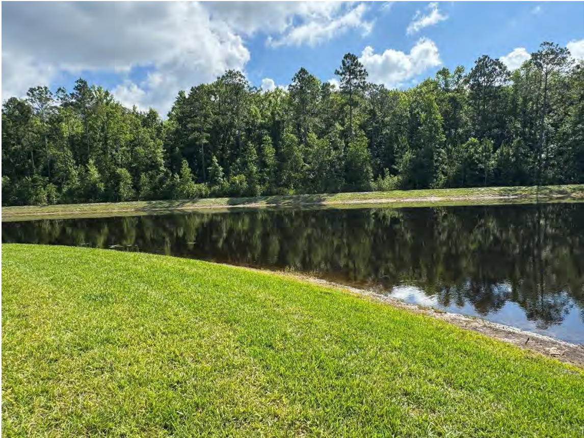
Beacon Lake Phase 1 – Storm Water Management Facility 3 (05-21-2026)
