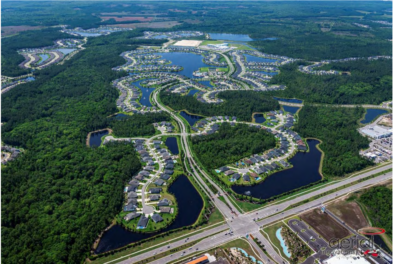
Beacon Lake – Aerial (By Aerial Innovations) (05-15-2025)
