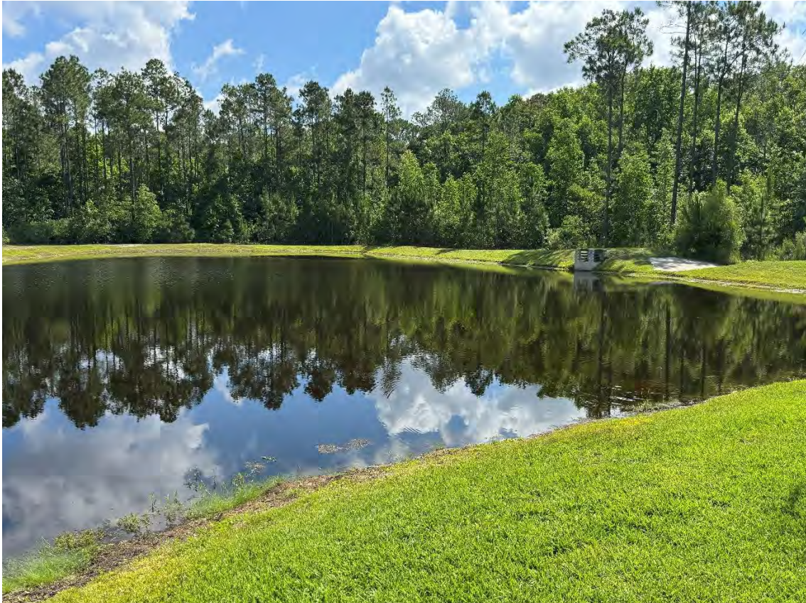
Beacon Lake Phase 1 – Storm Water Management Facility 4 (05-21-2026)
