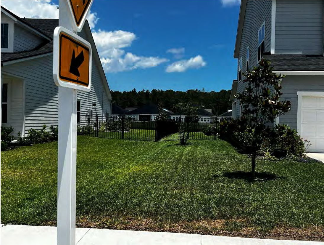
Beacon Lake Phase 4 – SMF 24 Easement Inaccessible due to Fencing (05-21-2026)
