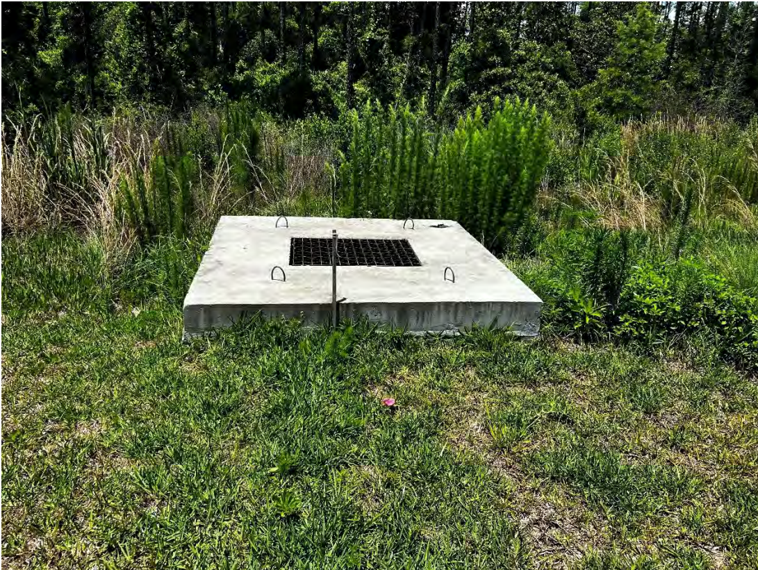
Beacon Lake Phase 4 – SMF 25 Control Structure (05-21-2026)
