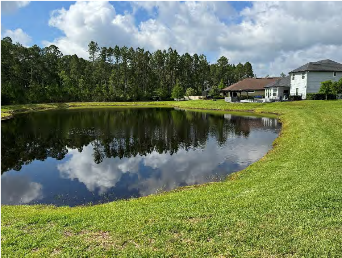
Beacon Lake Phase 1 – Storm Water Management Facility 13 (05-21-2026)
