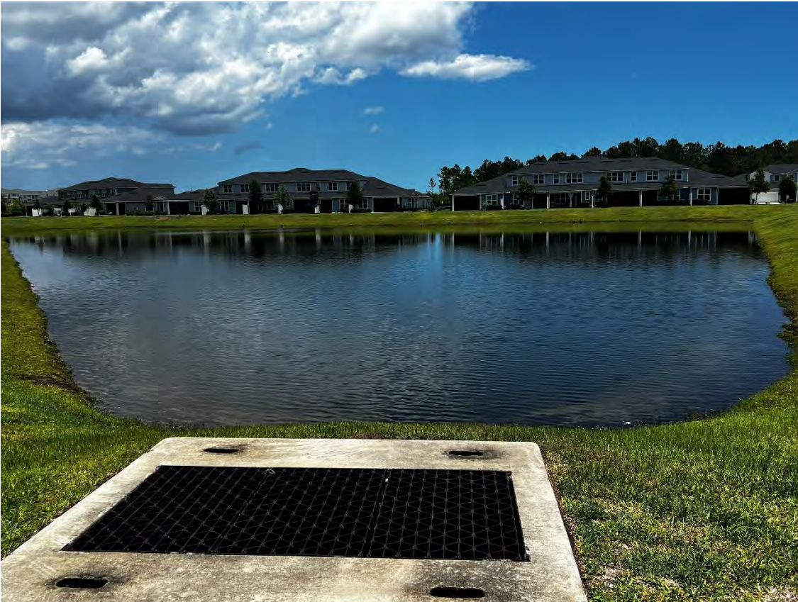
Beacon Lake Townhomes – Storm Water Management Facility 10 (05-21-2026)
