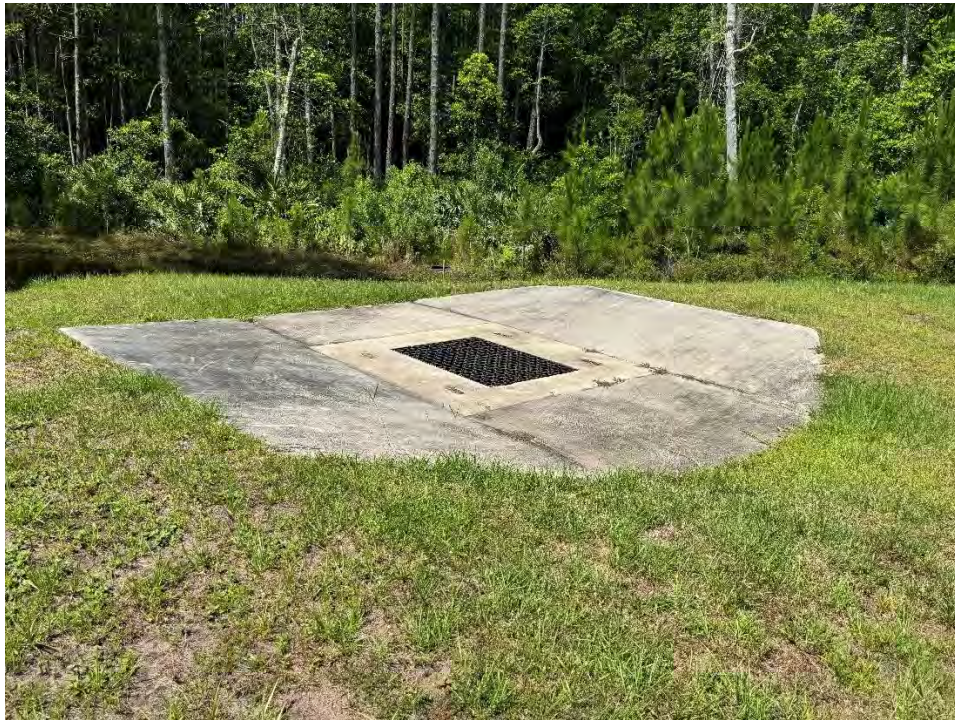
Beacon Lake Phase 2C – SMF 19 Control Structure (05-21-2026)
