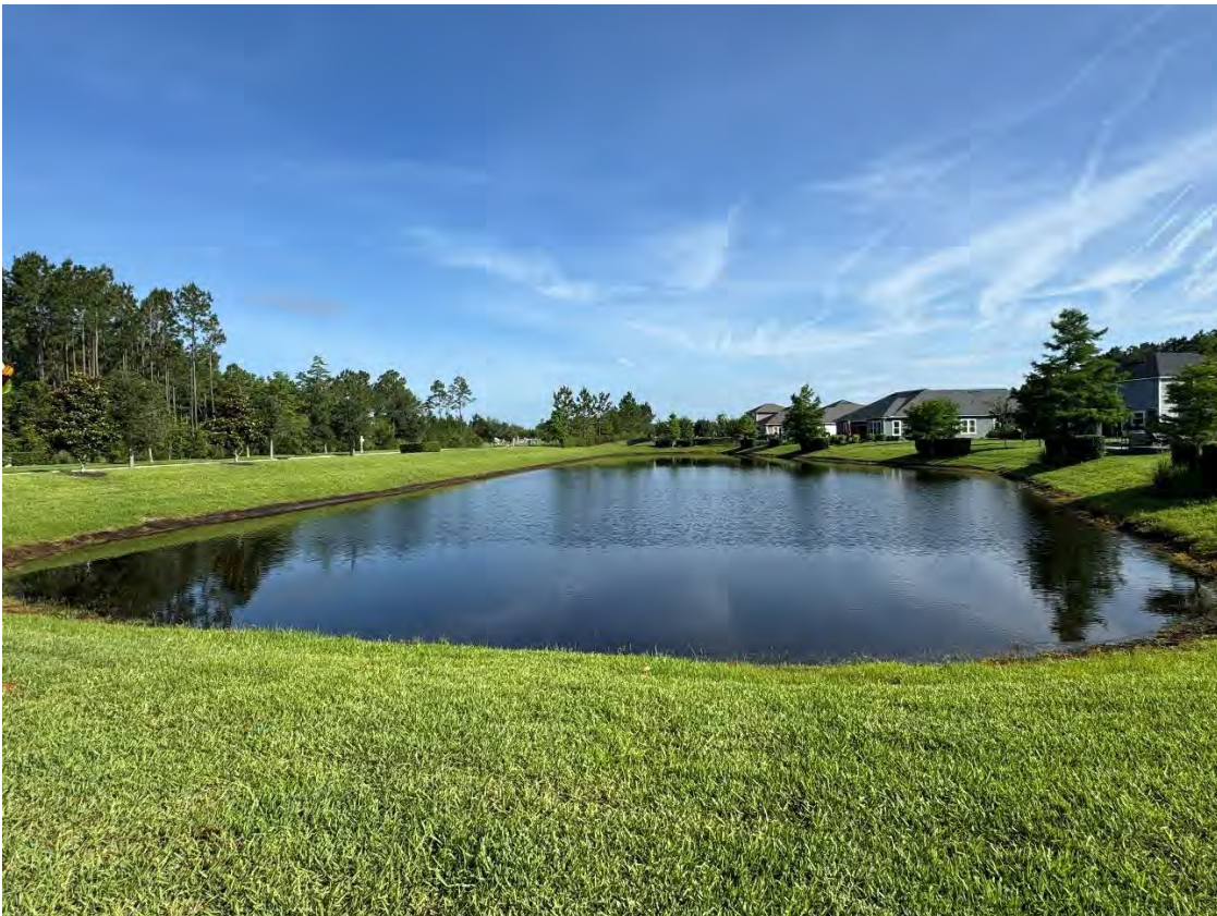
Beacon Lake Phase 1 – Storm Water Management Facility 2 (05-29-2026)
