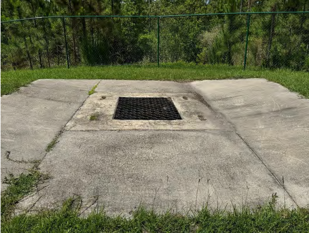
Beacon Lake Phase 2C – SMF 20 Control Structure (05-21-2026)
