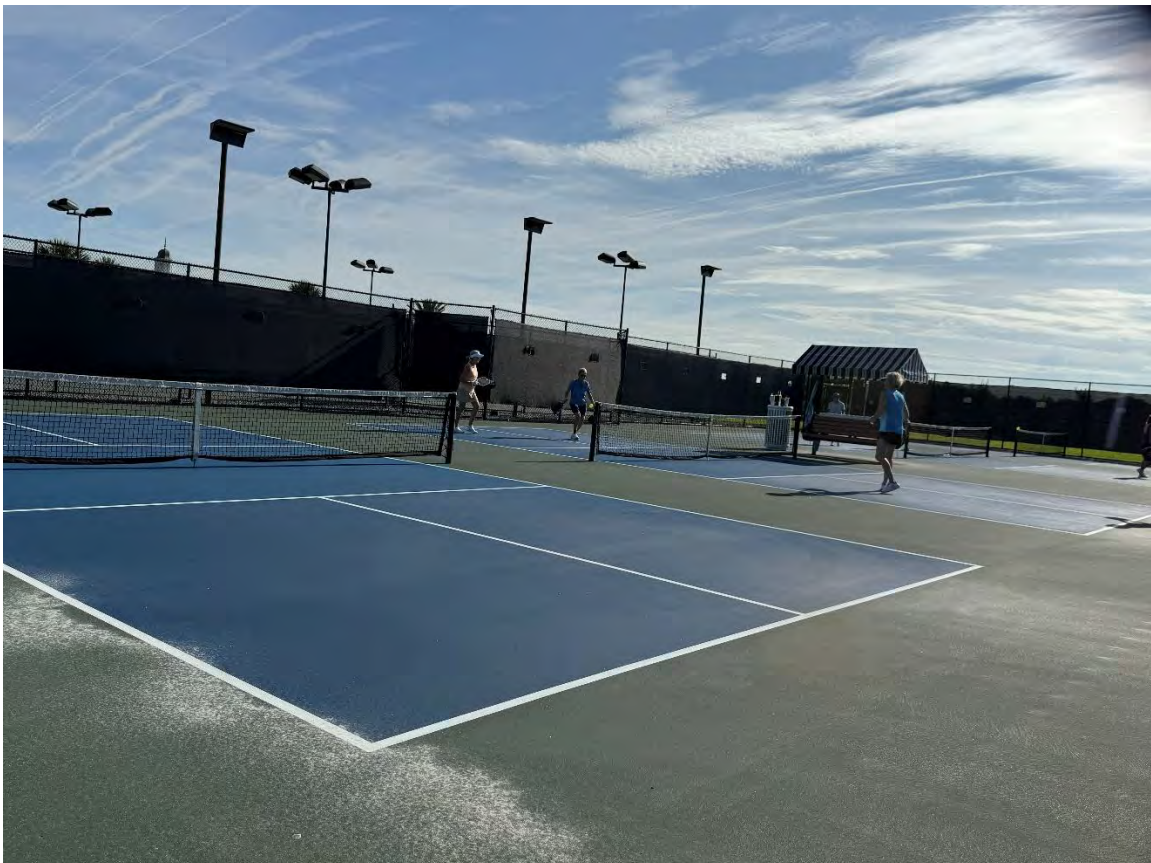
“Lake House” – Pickleball Courts (05-29-2026)
