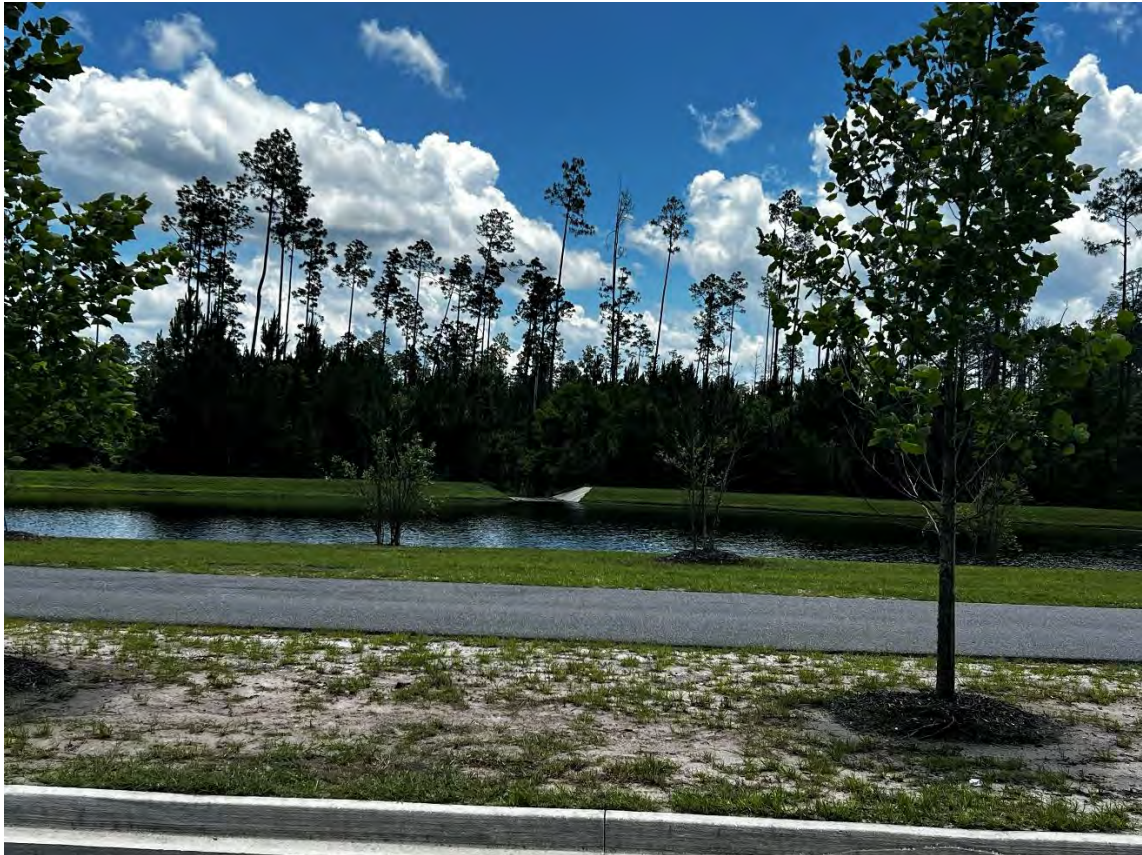
Beacon Lake Phase 1 – SMF 12 and 28 Control Structure (05-21-2026)
