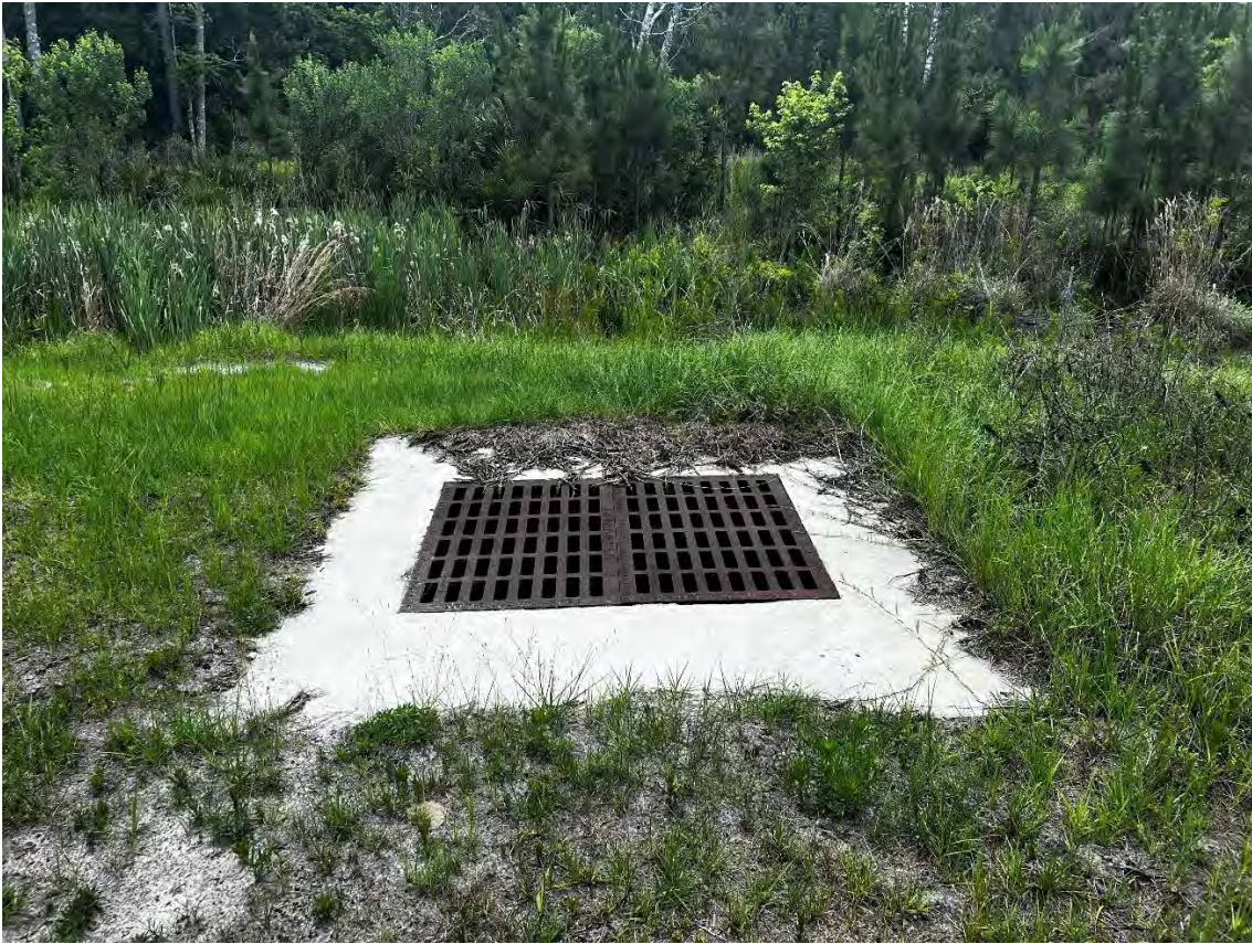
Beacon Lake Phase 3B – SMF 22 Control Structure (05-21-2026)
