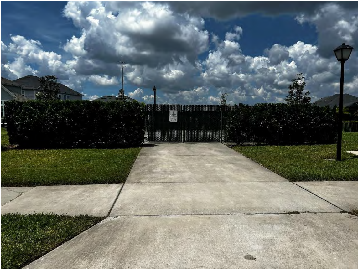
Loosestrife Way Lift Station (05-21-2026)
