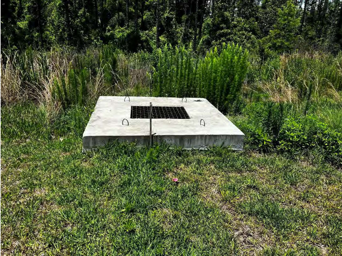
Beacon Lake Phase 4 – SMF 25 Control Structure (05-21-2026)
