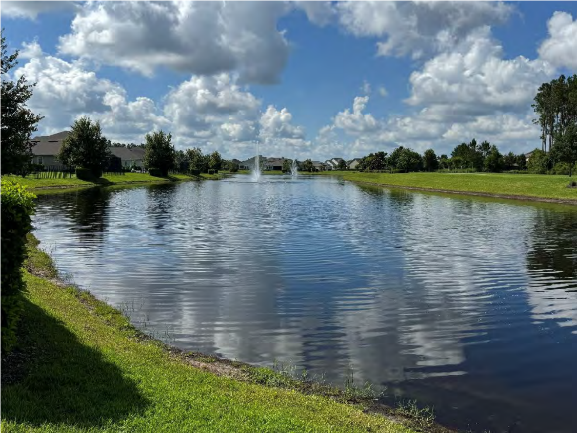
Beacon Lake Phase 1 – Storm Water Management Facility 5 (05-21-2026)
