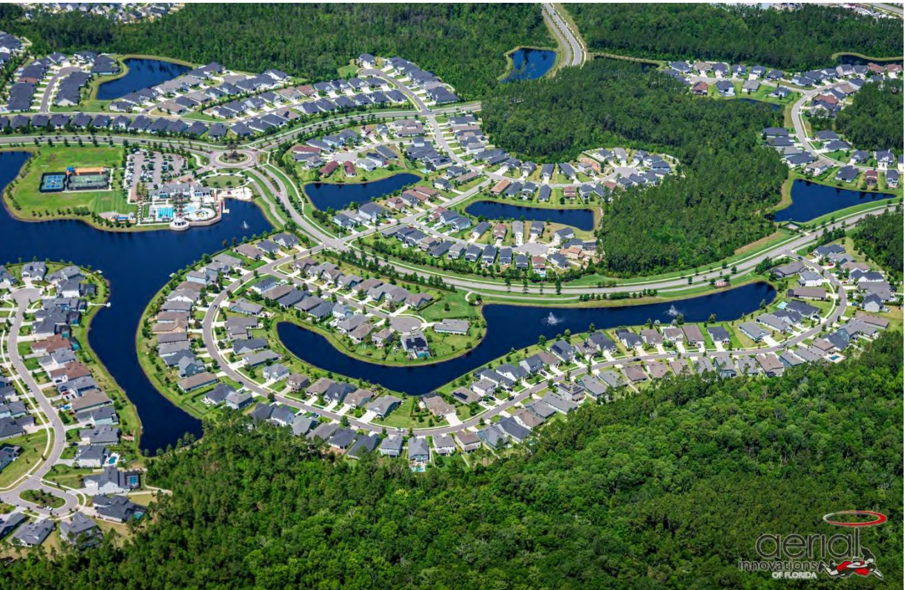
Beacon Lake Phase 1 – Aerial (By Aerial Innovations) (05-15-2025)
