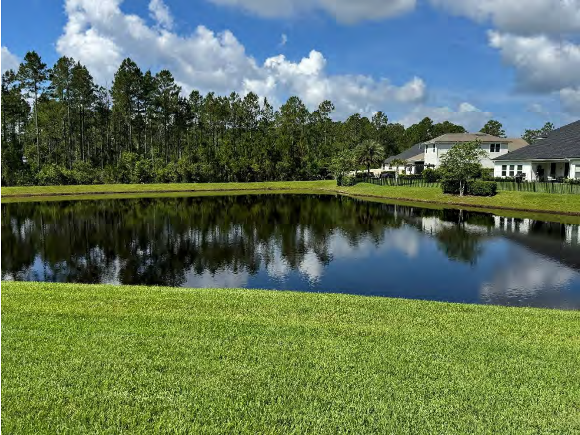
Beacon Lake Phase 1 – Storm Water Management Facility 14 (05-21-2026)
