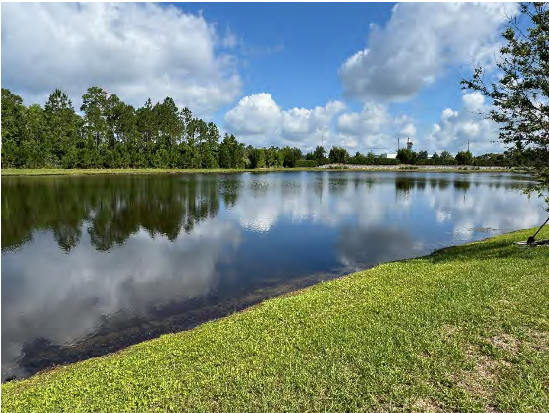
Beacon Lake Phase 1 – Storm Water Management Facility 11 (05-21-2026)
