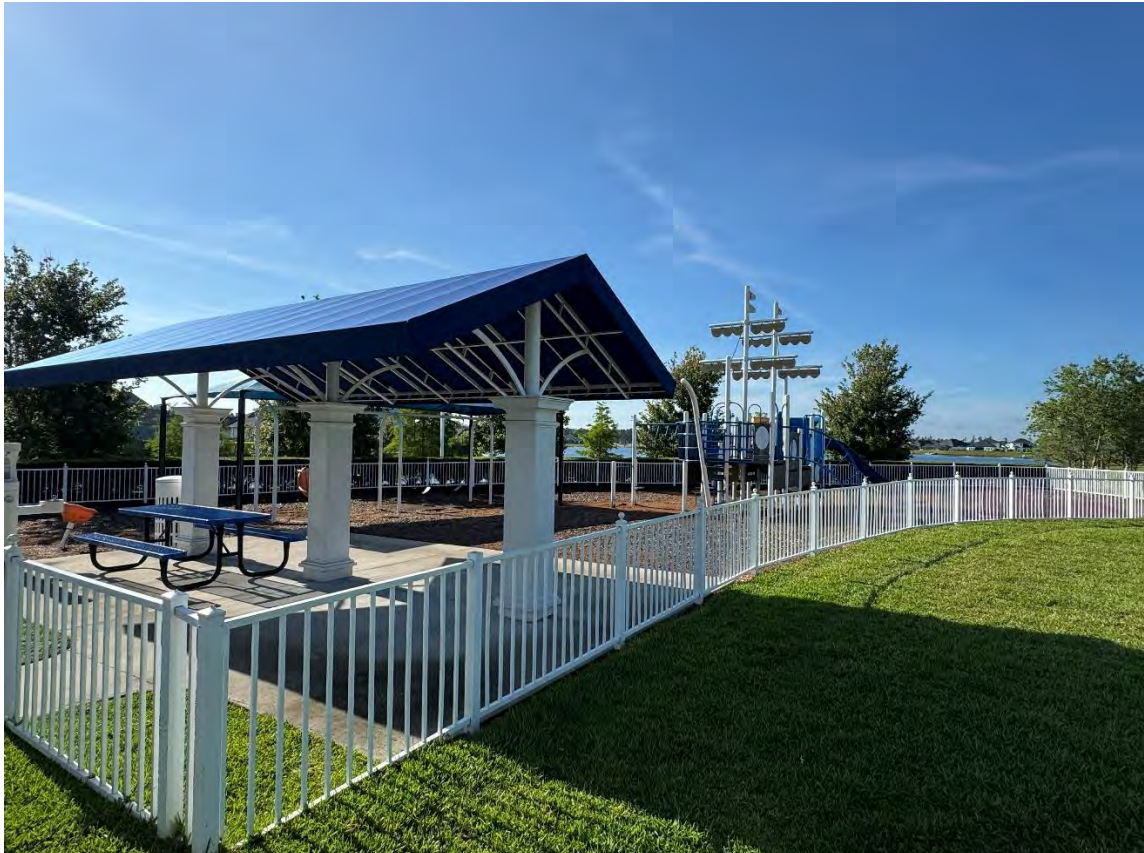
"Lake House" – Playground (05-21-2026)
