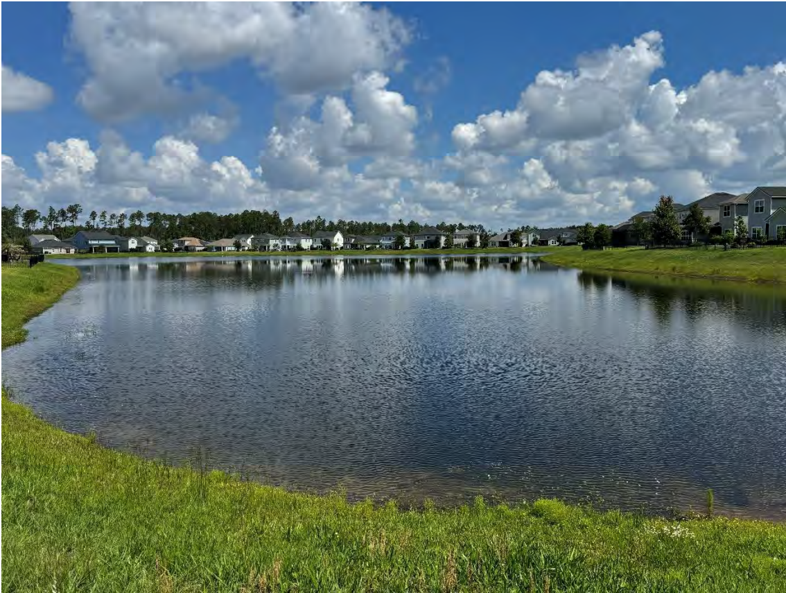
Beacon Lake Phase 2B – Storm Water Management Facility 18 (05-21-2026)
