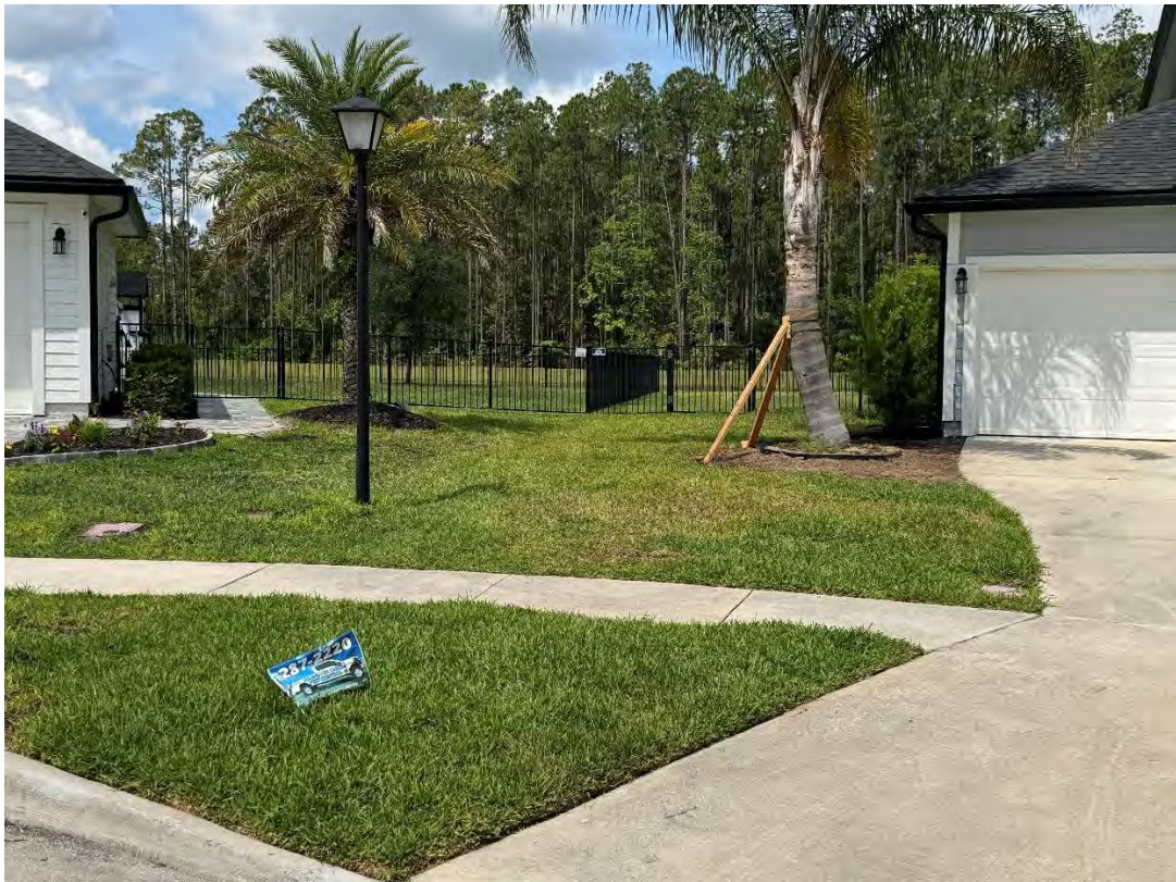
Beacon Lake Phase 2C – SMF 20 Easement Inaccessible due to Fencing (05-21-2026)
