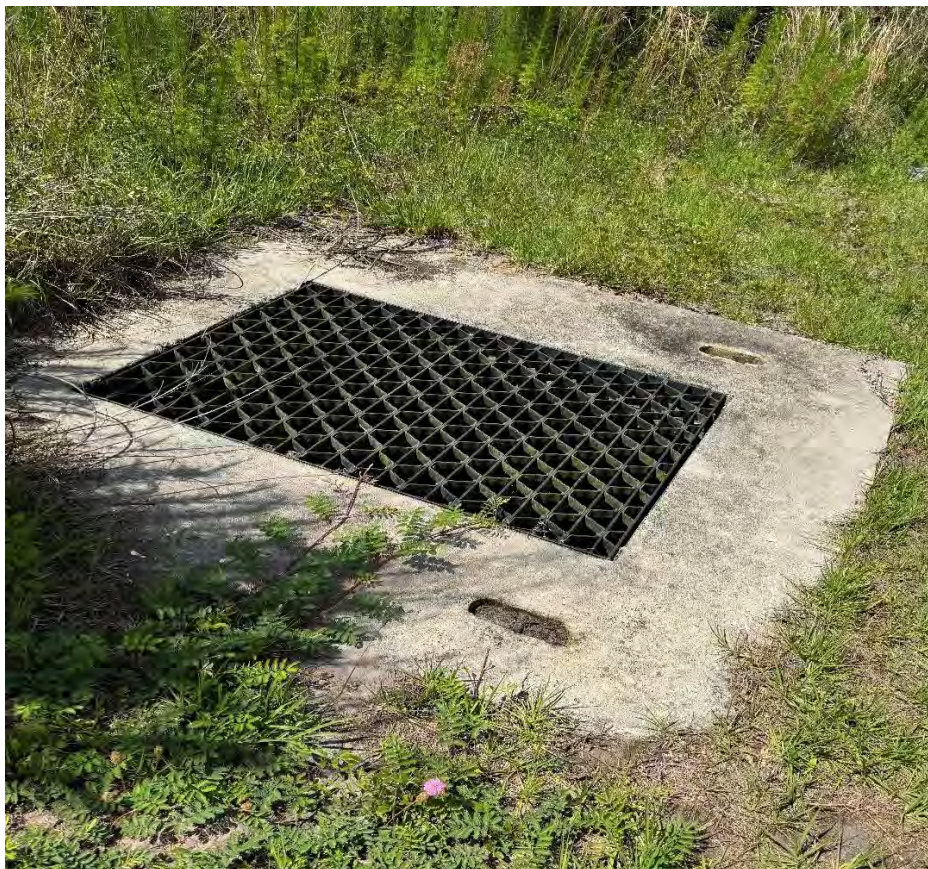
Beacon Lake Phase 2B – SMF 18 Control Structure (05-21-2026)
