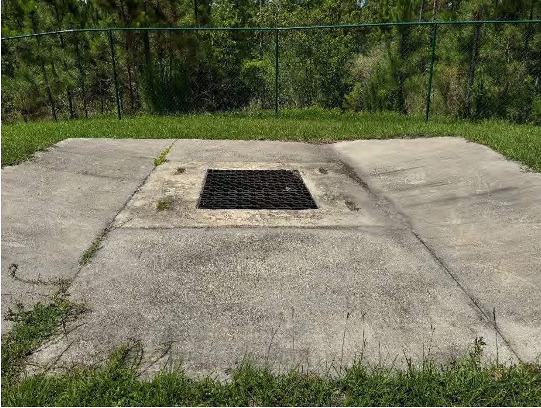
Beacon Lake Phase 2C – SMF 20 Control Structure (05-21-2026)
