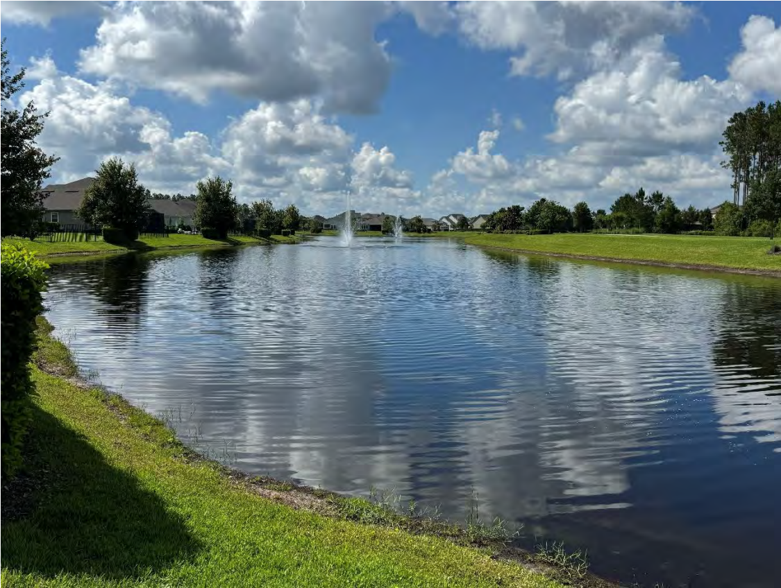
Beacon Lake Phase 1 – Storm Water Management Facility 5 (05-21-2026)
