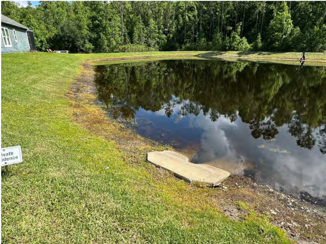
Beacon Lake Phase 1 – Storm Water Management Facility 3 (05-21-2026)
