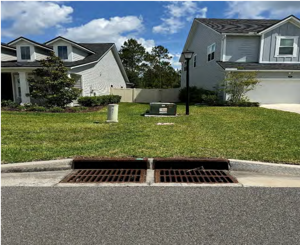
Beacon Lake Phase 2B – SMF 18 Easement Inaccessible due to Fencing (05-21-2026)
