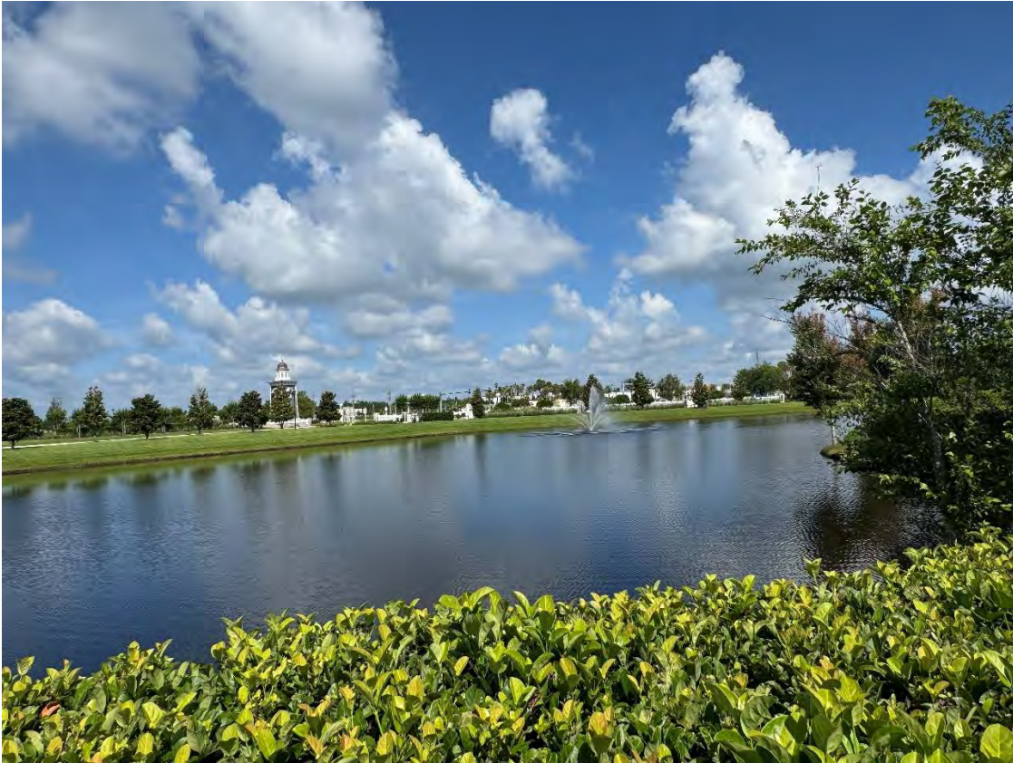
Beacon Lake Phase 1 – Storm Water Management Facility 1 (05-21-2026)
