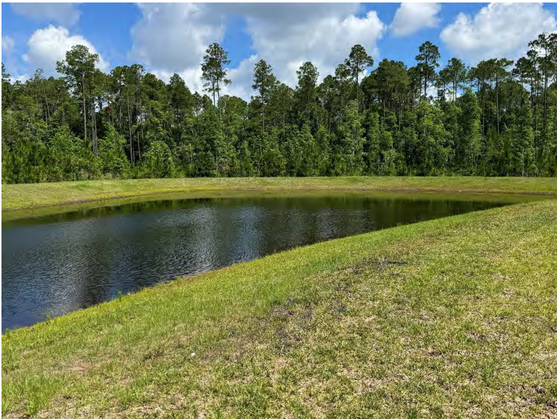
Beacon Lake Phase 2C – Storm Water Management Facility 19 (05-21-2026)
