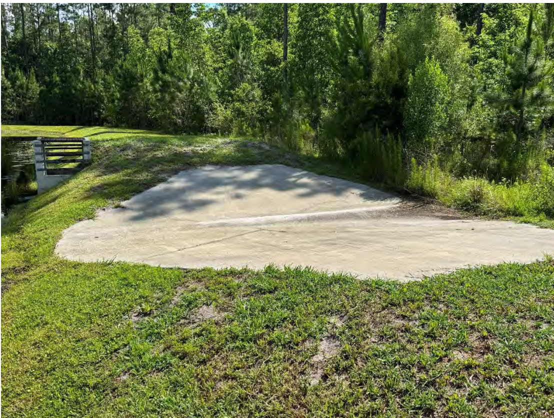
Beacon Lake Phase 1 – SMF 4 Spillway and Control Structure (05-21-2026)
