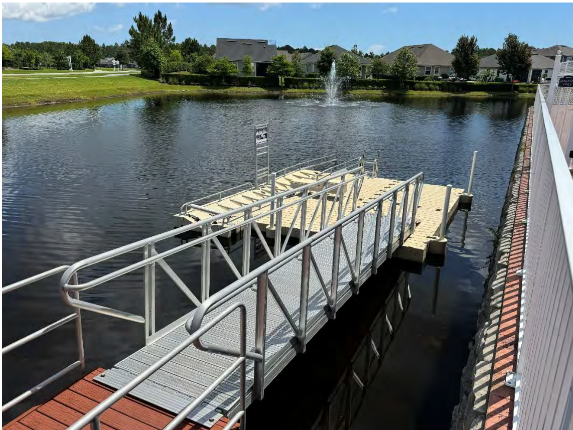
Beacon Lake Phase 1 – Storm Water Management Facility 6 (05-21-2026)
