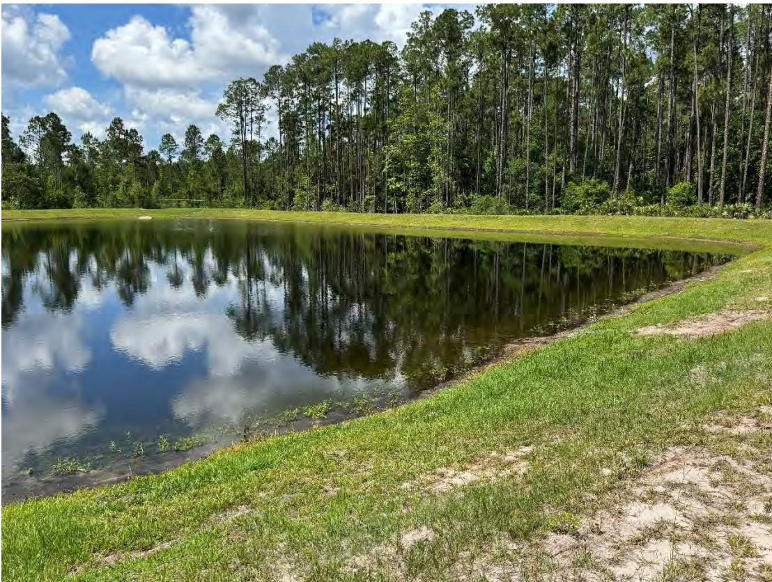
Beacon Lake Phase 2C – Storm Water Management Facility 20 (05-21-2026)
