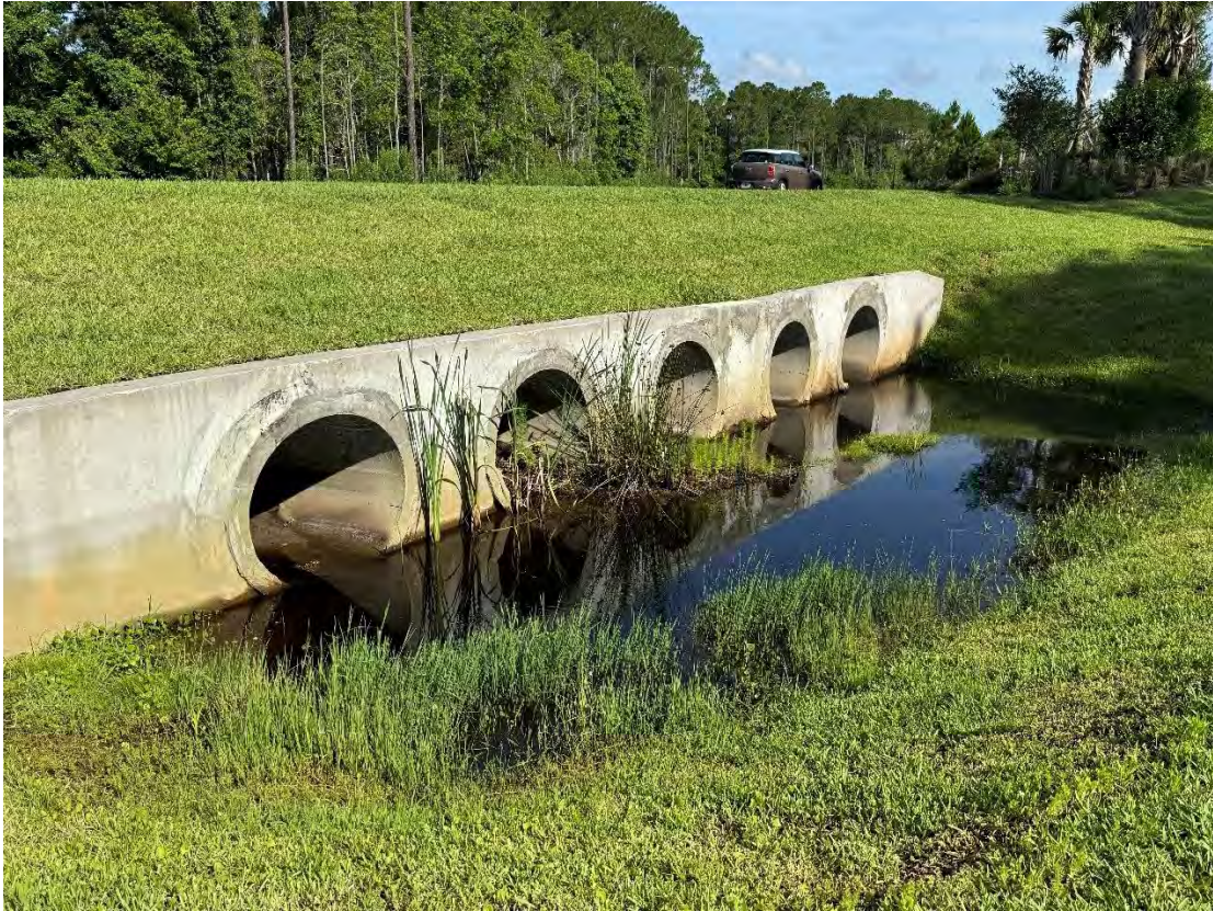
Beacon Lake Phase 4 – Cross drains on Heron Oaks Drive (05-29-2026)
