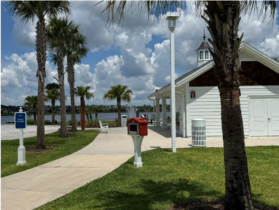
Beacon Lake Phase 3A Lakeside Park (05-29-2026)
