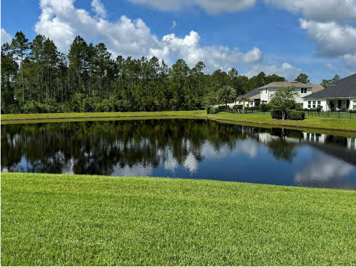
Beacon Lake Phase 1 – Storm Water Management Facility 14 (05-21-2026)
