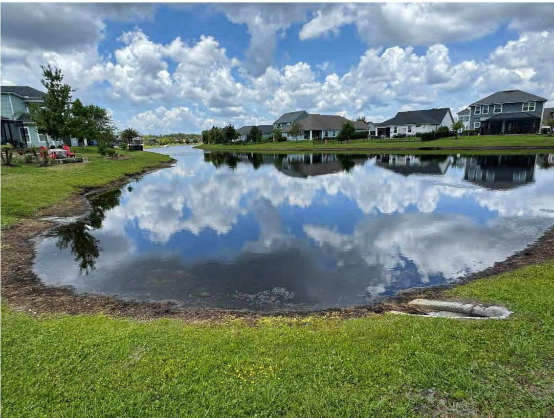
Beacon Lake Phase 3A – SMF 6 Outflow Structure (05-21-2026)
