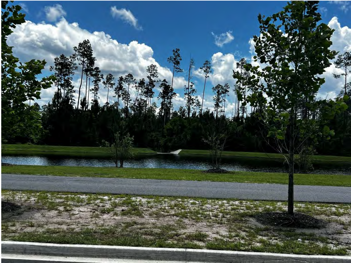
Beacon Lake Phase 1 – SMF 12 and 28 Control Structure (05-21-2026)
