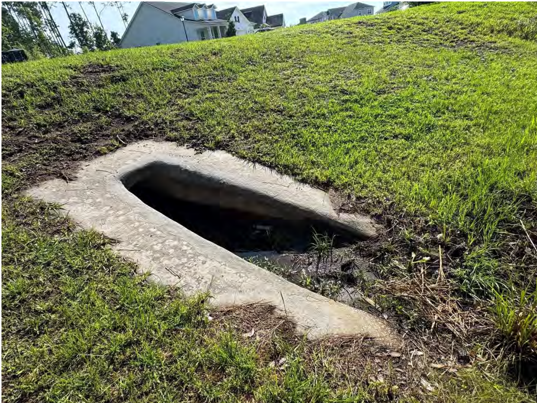
Beacon Lake Phase 2C – Cross drain on Windermere Way (05-29-2026)
