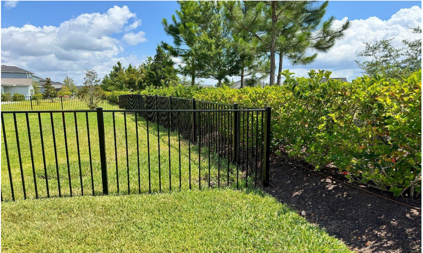
Beacon Lake Phase 2 – Obstructed Drainage and Access Easement for lots
