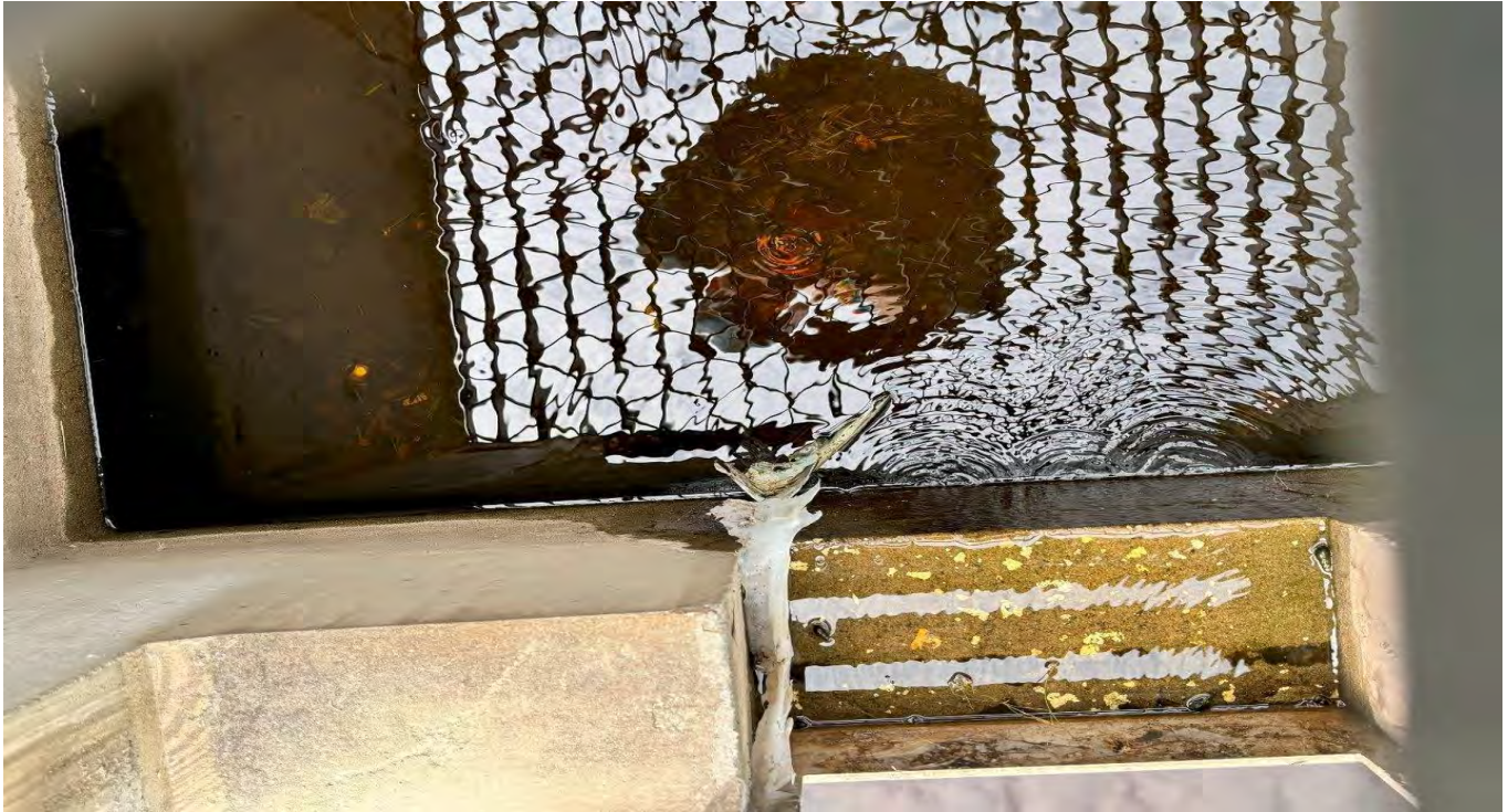
Beacon Lake Phase 1 – Storm Water Management Facility Control Structure 11 Weir Plate Leaking (06-07-2024)
