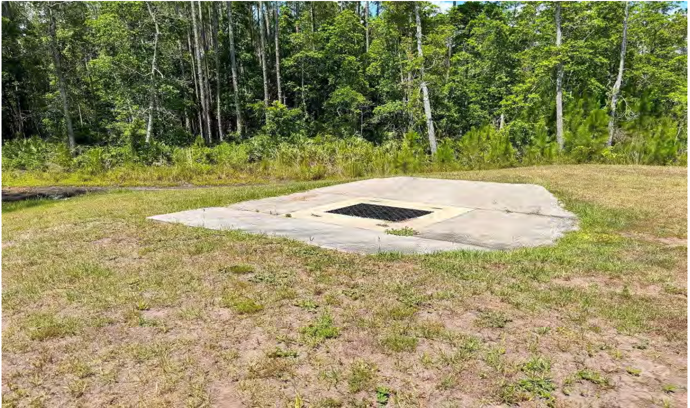
Beacon Lake Phase 1 – Storm Water Management Facility Control Structure 19 (06-07-2024)
