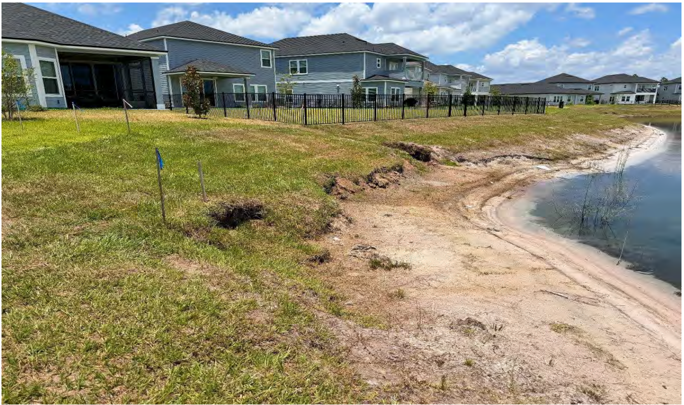
Beacon Lake Phase 3B – Erosion Concerns at Storm Water Management Facility 22 (06-07-2024)
