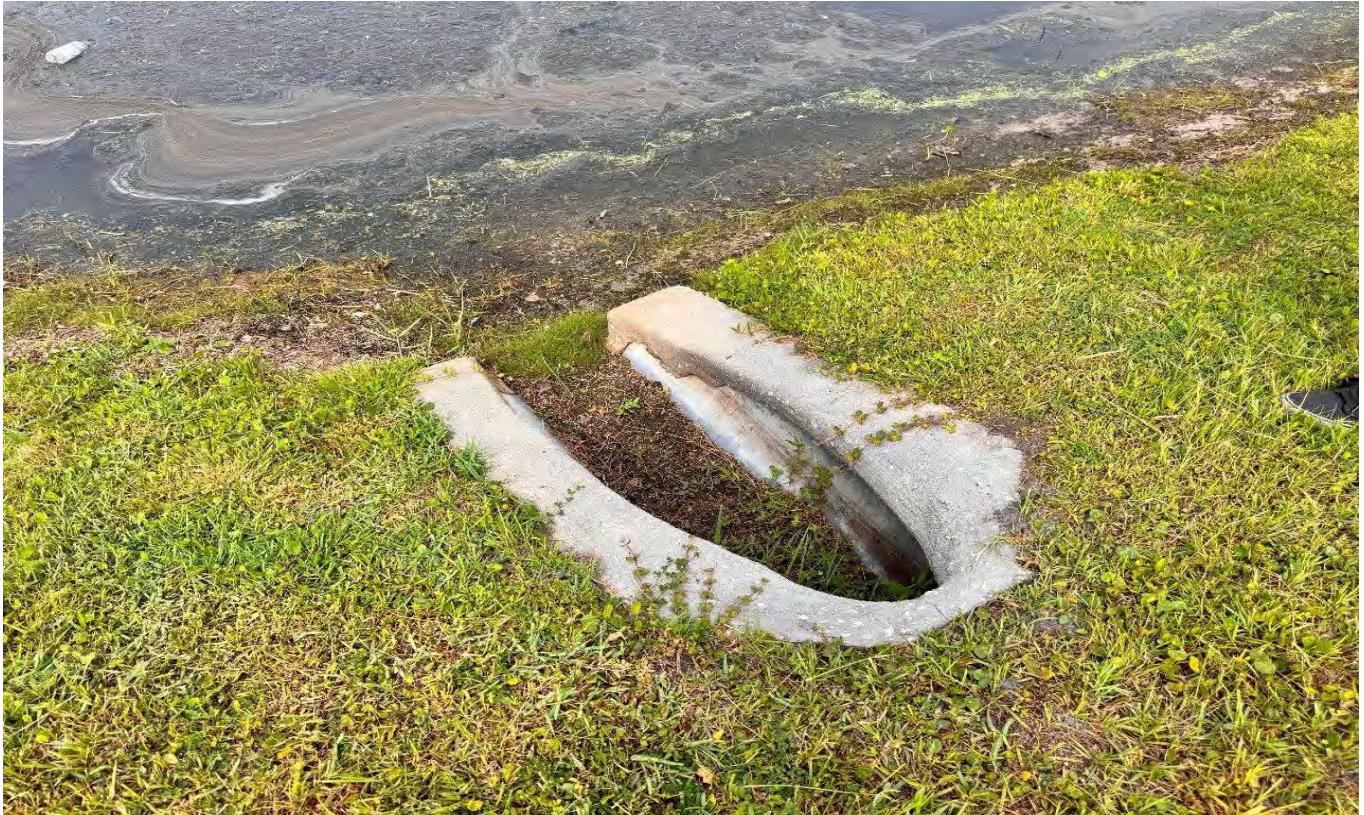
Beacon Lake Phase 1 – Storm Water Management Facility 6 Emergency overflow pipe (06-07-2024)
