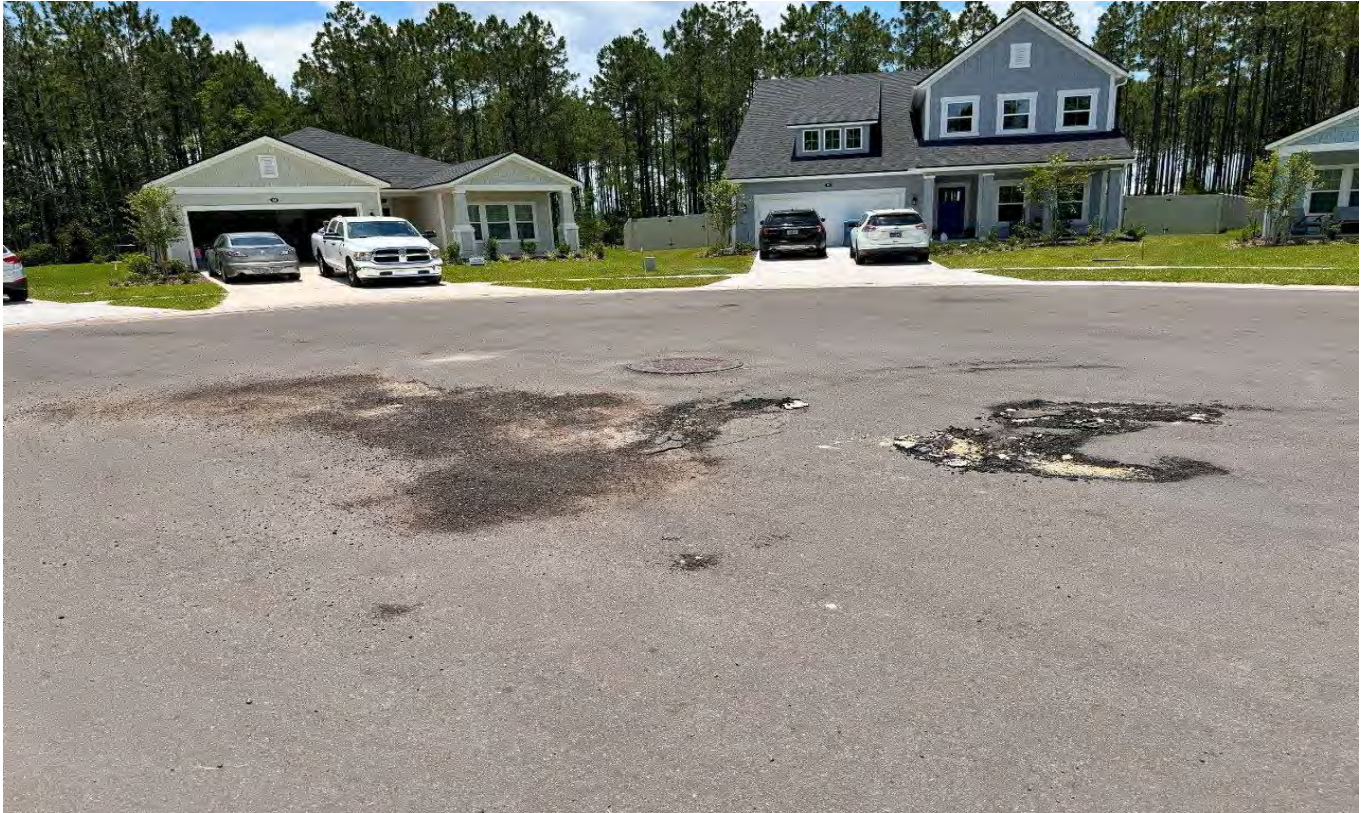
Beacon Lake Phase 4 – Exposed Lime Rock and Damaged Pavement along Wetland Avenue (06-07-2024)
