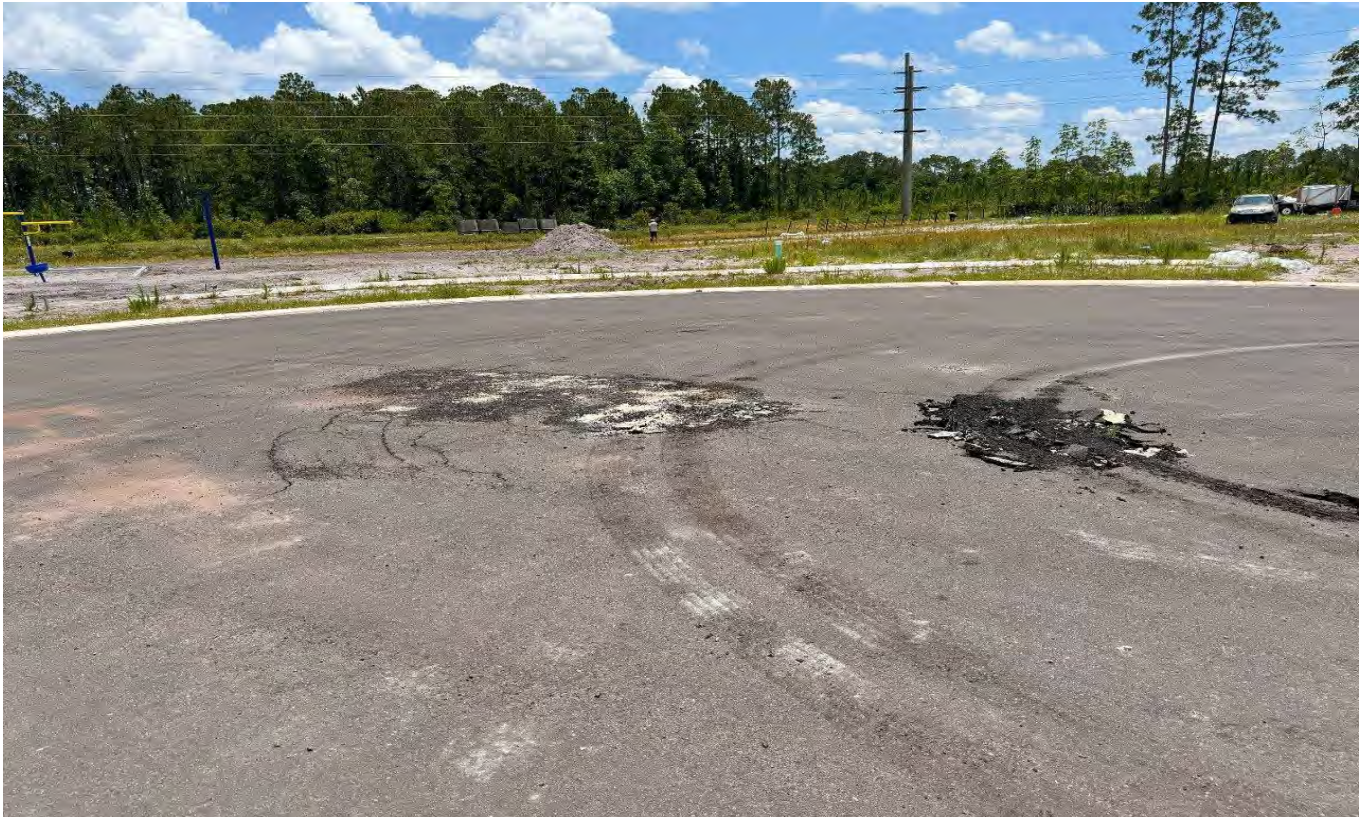
Beacon Lake Phase 4 – Exposed Lime Rock and Damaged Pavement along Quiet Wharf Drive (06-07-2024)
