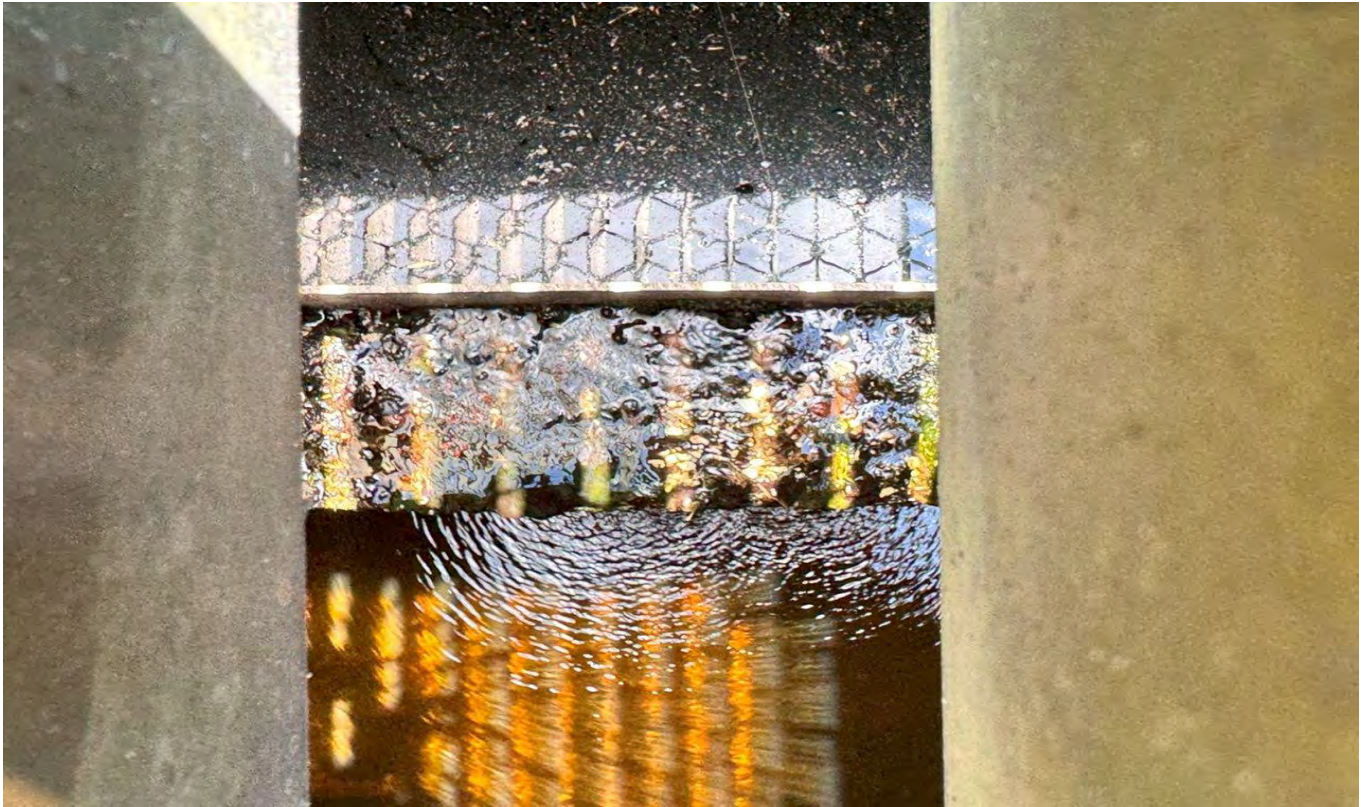
Beacon Lake Phase 2 – Storm Water Management Facility Control Structure 18 Weir Plate Leaking (06-07-2024)
