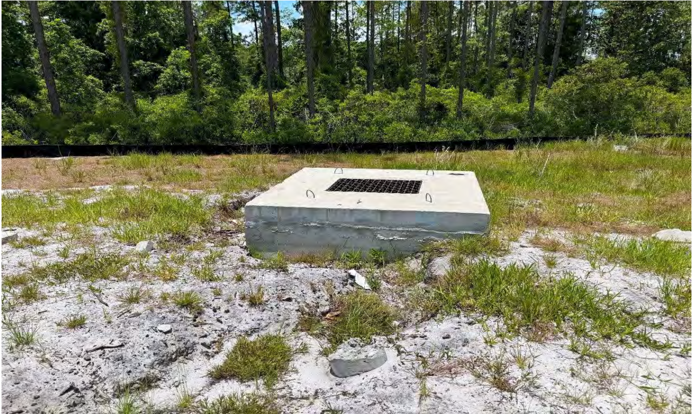
Beacon Lake Phase 4 – Storm Water Management Facility 25 Control Structure (06-07-2024)
