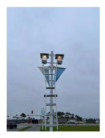
Five LED lights and ballast were replaced on the tall white poles.
