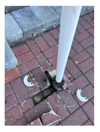
Loose railings were repaired with cement.
