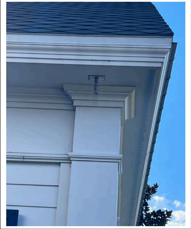
Photo sensor was replaced with a different style that allows more light in so the lights turn off sooner.
