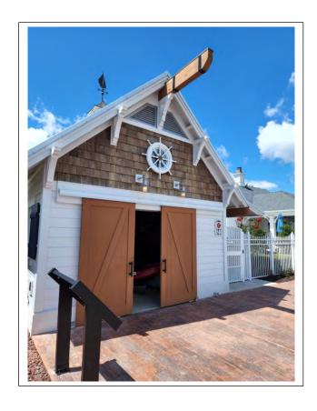
Cedar shingles on the kayak house were pressure washed and are currently being sealed with a transparent water sealer
