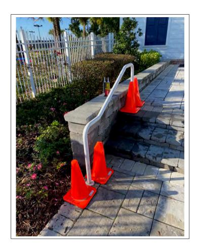
A handrail on the pool deck was repaired by recementing it into the pavers
