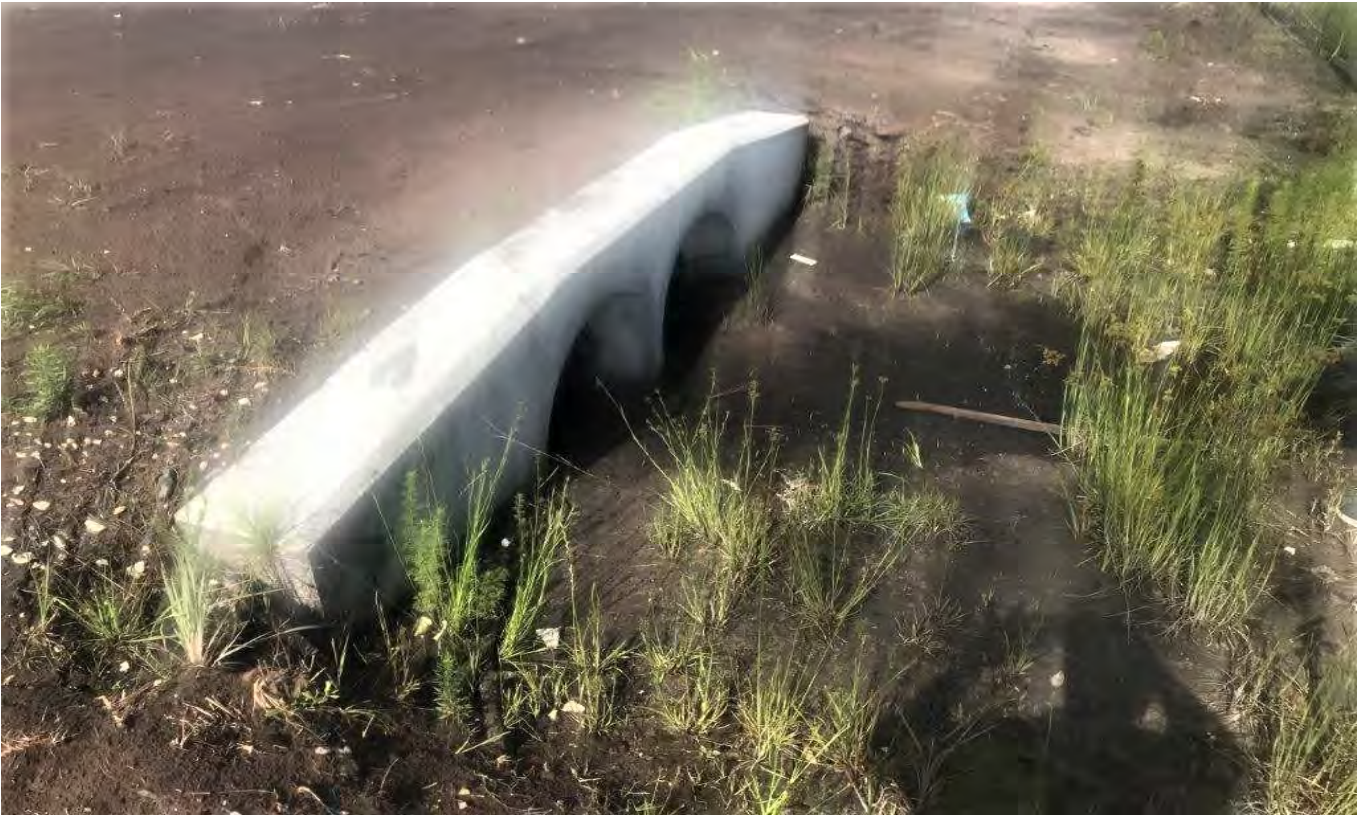
Culvert Equilizer structure (Hutchinson Lane) (5-7-2019)
